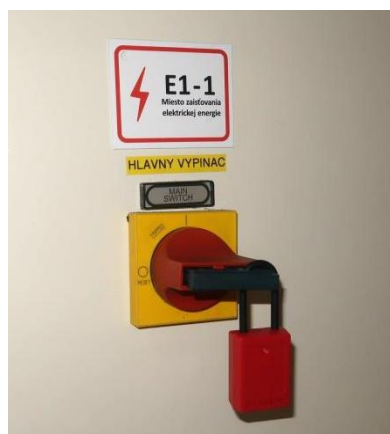
Fig. 1 Example of hazardous electric energy isolation
